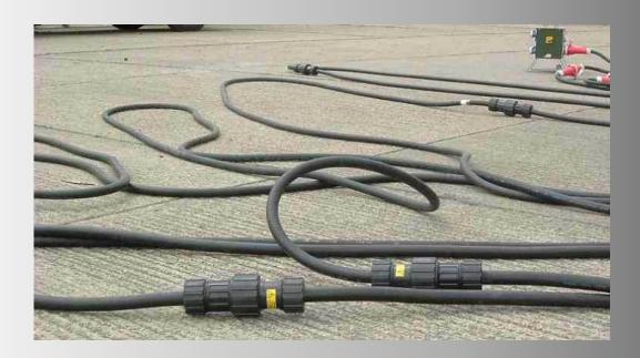
LUGIT is a safe and efficient means to make temporary connection / extensions of single core power cables that are pre-terminated with copper lug terminals.
